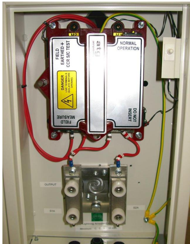
Figure 7-1 Cutout Switch mounted in CCR HT Output Terminal box
