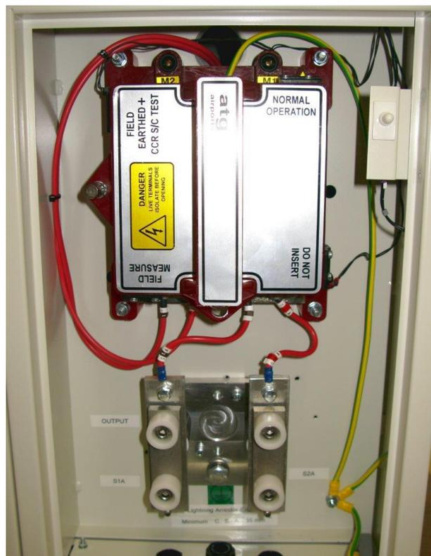
Figure 6-1 Cutout Switch mounted in CCR HT Output Terminal box
