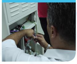
The new Micro100 Constant Current Regulators (CCR's) being installed to power the addition circuits, employ dual redundant profibus interface which therefore requires the existing network to be extended in each of the substations. Software modification to control each application, taxiway routes and stobars, were coded and uploaded. The graphical representation of the airfield layout was amended to reflect the new taxiway layout, along with the new hardware being included on substation diagrams.
