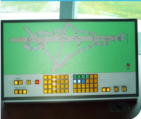
Although the control system over the years had several modifications to accommodate new services, very little had changed with the overall system. However, the mimic panels had over time, lost their shine, and TAG Aviation contracted atg airports to upgrade the system for the use of, the now accepted, 'touch screen control panels'
