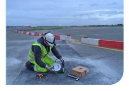
Within the substations there was a requirement to add new power supply feeds for the additional constant current regulators selected from the Micro200 range of CCR's, along with associated supply breakers. New stopbar fixtures were installed on the taxiway routes along with, taxiway centreline lighting, utilising the IR range of LED lighting fixtures. The Clearway brand of LED taxiway guidance signs were installed, along with the Apollo runway guard lights.
